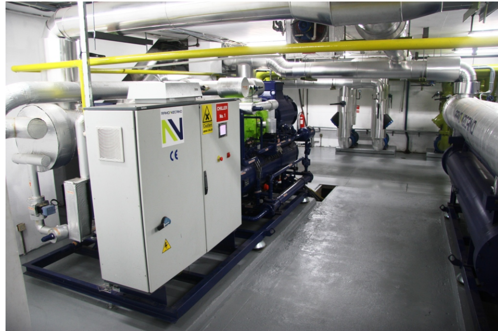
Ammonia Chiller AC Installation / Basement Public Building
